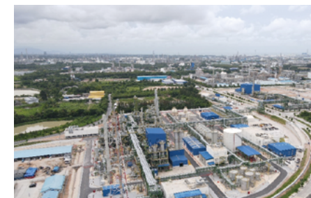
Aerial view of the new plant
